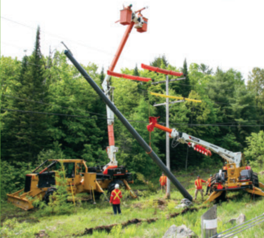
An AD610C equipped with a digger derrick holds the new pole in place.
