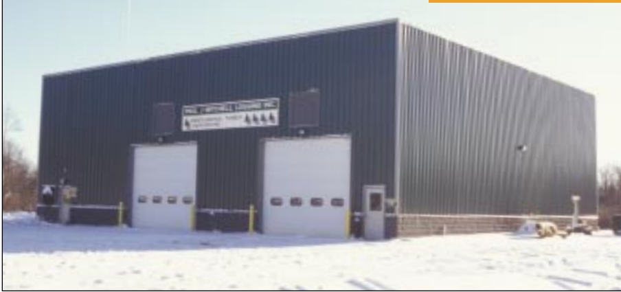
Mitchell's new 6,400 sq. ft. shop and office facility.
