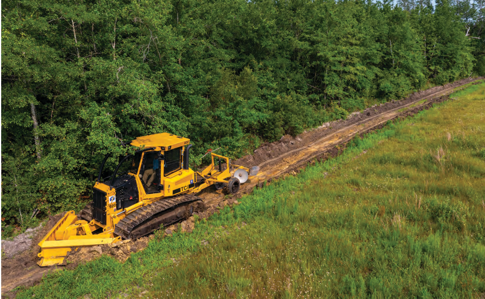
On the second pass, the V-blade clears any remaining debris, widens the break, and grades the surface to allow for vehicle access.
