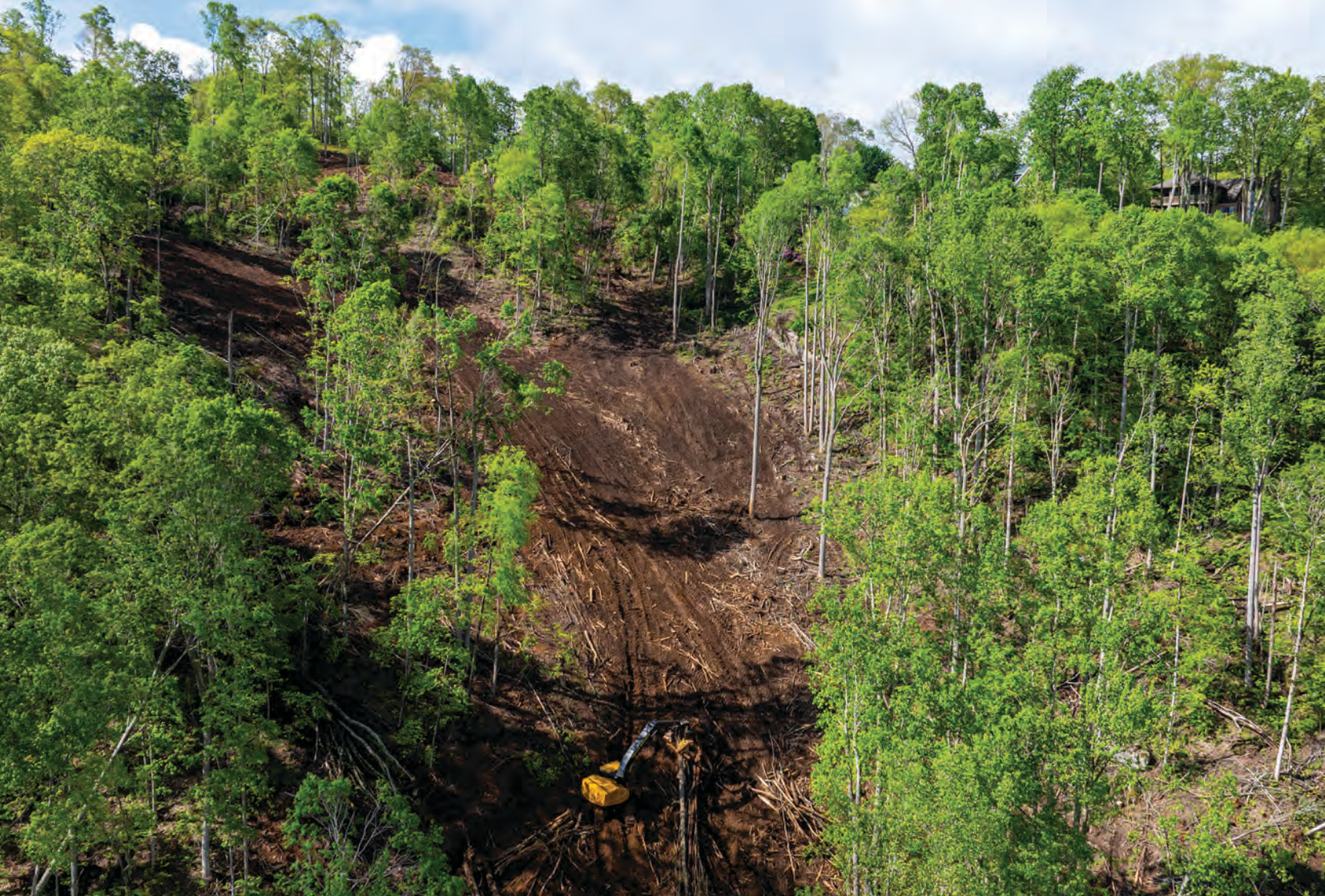
A challenging worksite. Chase believes the Tigercat LS857 is the best solution to safely tackle this extreme terrain storm cleanup contract.
