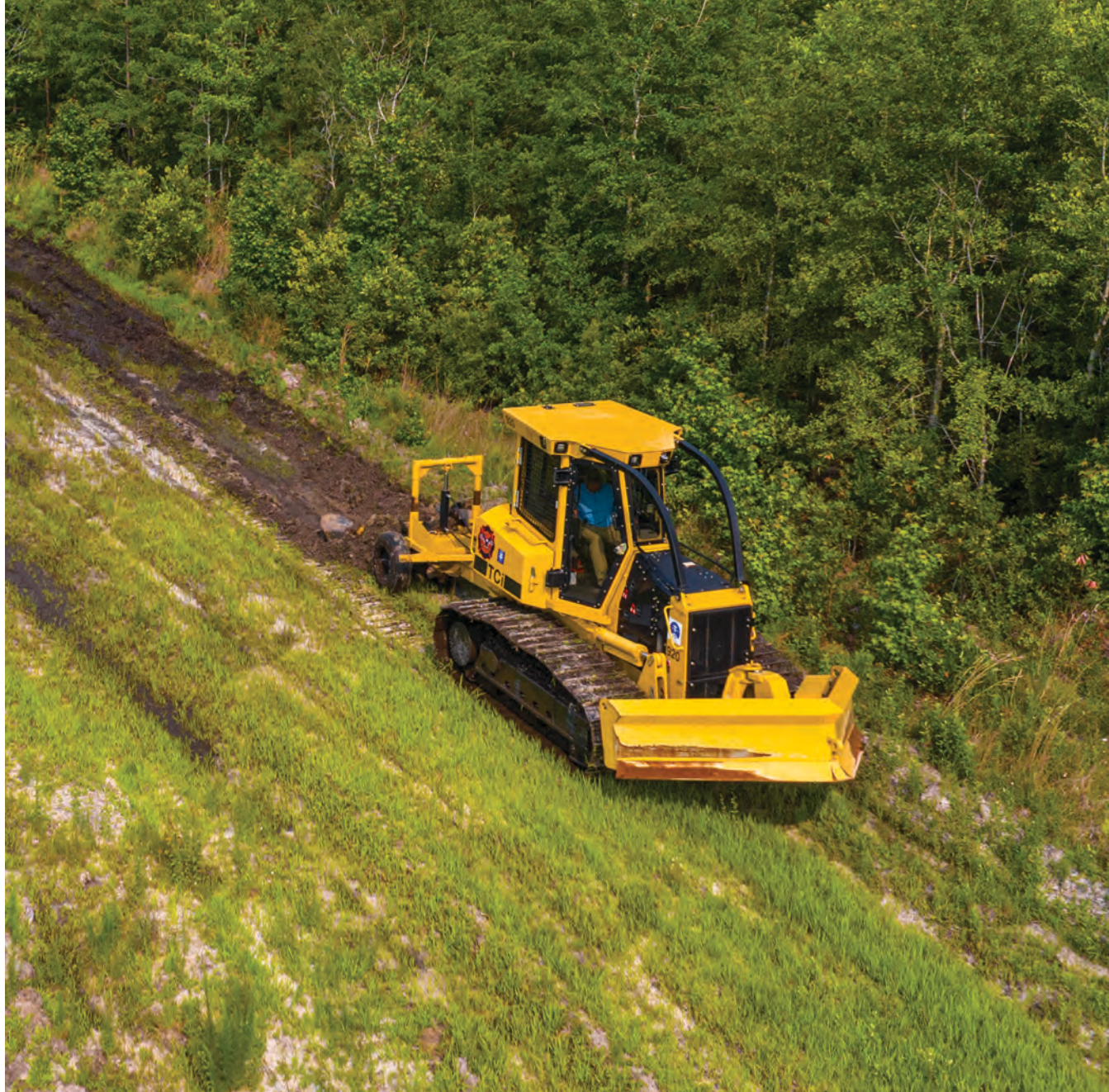
Chris makes a first pass on a perimeter firebreak with the plow engaged.
